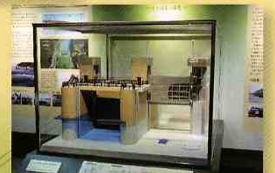
Model of gates of new main weir Model illustrating the complexities of the first submerged weir in Japan to have self-propelled hydraulic gates
