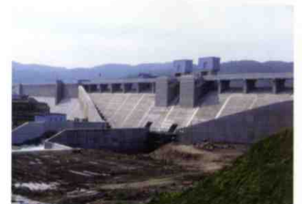
Pirika Dam completed in 1991
