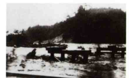
Inaho Bridge washed out during the flood in August 1929.
