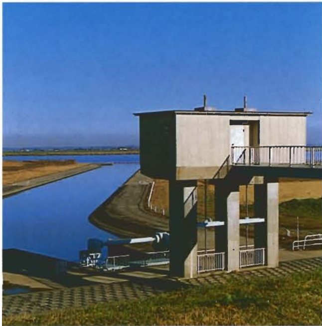
● Hokusotobu Canal (Intake structure)
