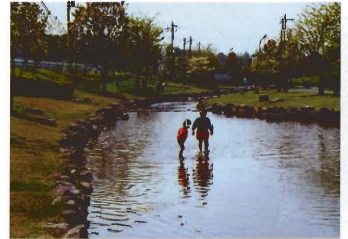
During the reconstruction of the Minumadai Irrigation Canal (Saitama Goguchi Project - Stage II), part of it was covered to create open spaces where local municipalities created waterside parks.
