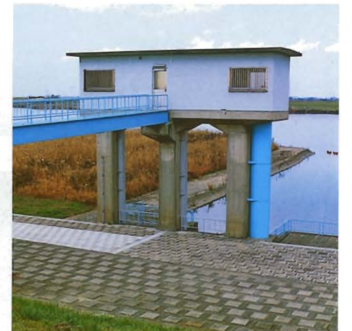
● Narita Canal (Intake structure)
