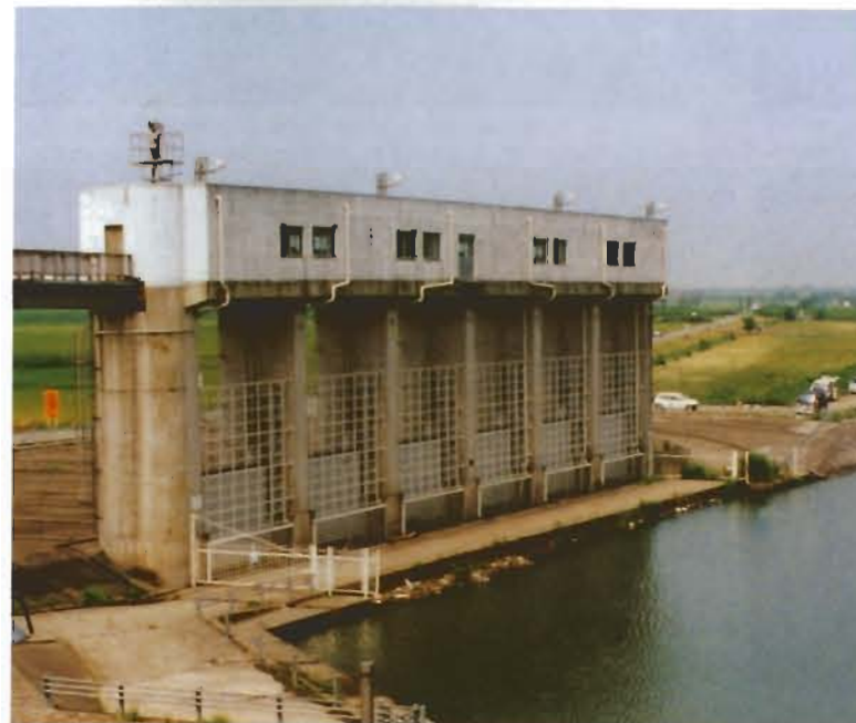
● Asaka Canal Reconstruction (Intake structure)
