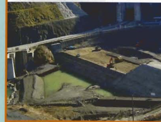
Upstream cofferdam for the Tokuyama Dam
