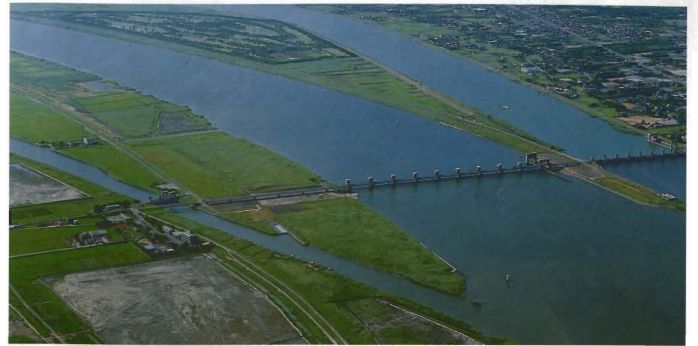
● Tonegawa Estuary Barrage
