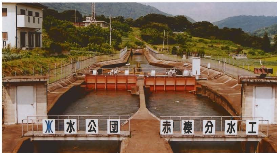
● Gunma Canal (the Tone River Aqueduct Bridge)
