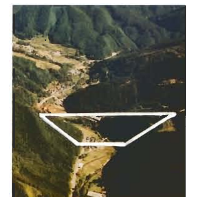
● Koishiwaragawa Dam (Dam Site)
