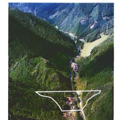
● Oyama Dam (Dam Site)
