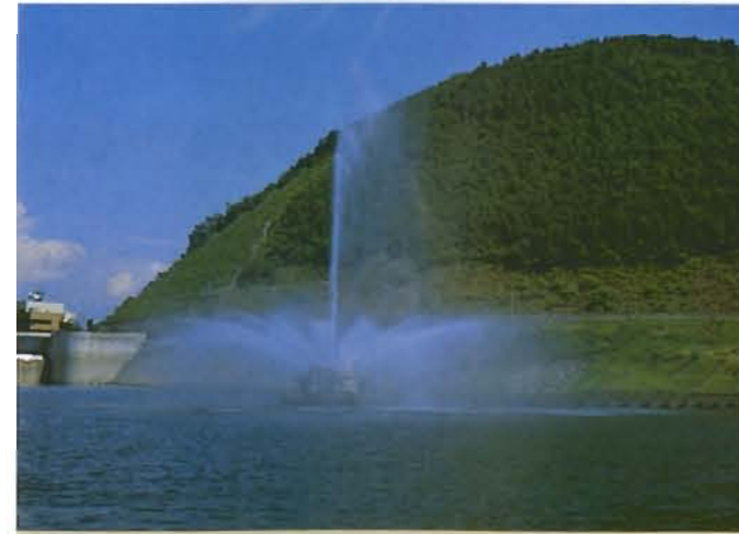
To conserve water quality, the Agigawa Dam incorporates a selective intake facility, check dams, shallow aeration facility (fountains), and many other devices.
