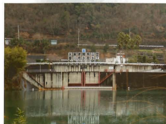
Kagawa Canal (Intake Structure)
