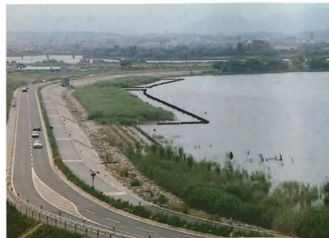
In the Lake Biwa Development, special care to protect reed fields was taken during the construction of lake bank levees and maintenance roads. Although part of the reed fields had to be ruined, compensation planting was carried out.
