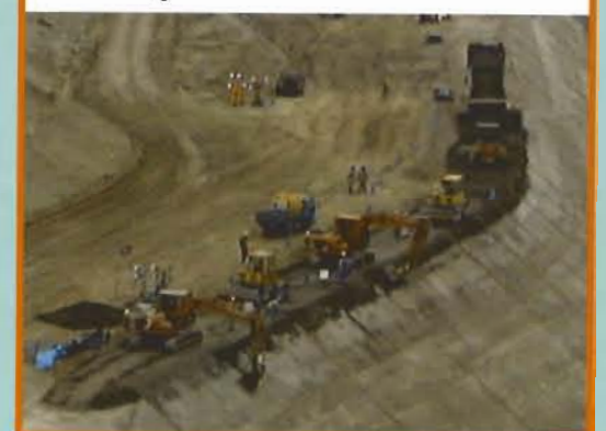
Counterweight embankment for the Takizawa Dam
