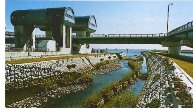
At the Nagara River Estuary Barrage, various types of fishways were created. The "rippling fishway" (above), designed with a gentle slope and natural pebbles, has been proven to be effective in allowing various fish species to migrate up and down the river. The "fishway with attraction flow (right)" is provided with a fishway observation room, in which visitors can view the fishes migrating up the river.
