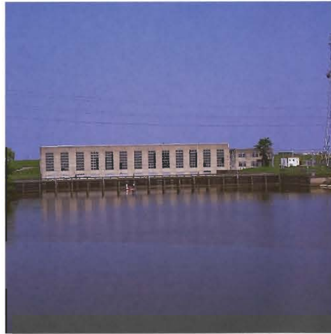
● Inbanuma Facilities Emergency Reconstruction Project (Inba Pumping Station)
