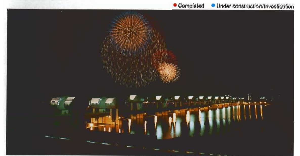
● Nagarakawa Estuary Barrage
