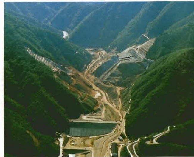
● Tokuyama Dam (viewed from the upstream side)
