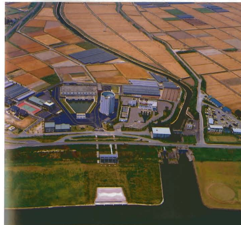
● Chikugogawa Karyu Canal (right-bank intake and Saga pumping station)
