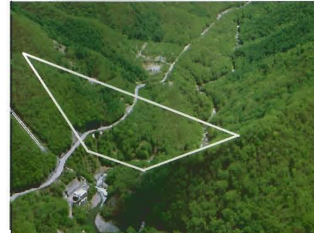
● Tokura Dam (Dam Site)
