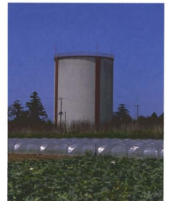
● Toso canal (Iioka Surge Tank)
