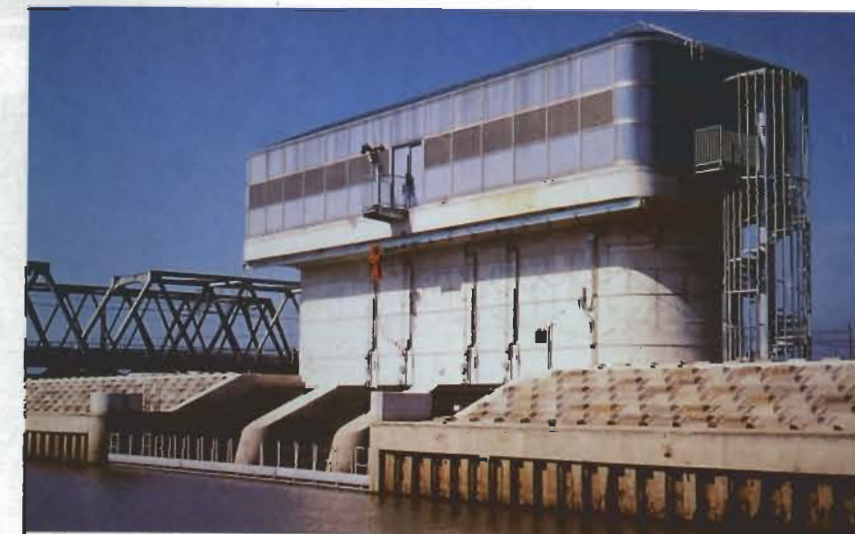
● Nagara Canal (Intake structure)
