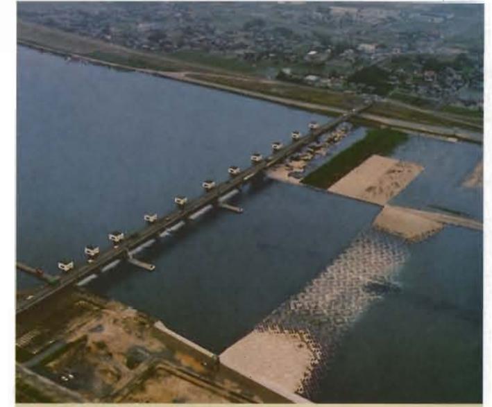
In the Tone Barrage Facilities Emergency Reconstruction, the ingenious shape of the barrage and the arrangement of streambeds protection allowed fish to travel upstream throughout the channels even when the water level changed during the work.
