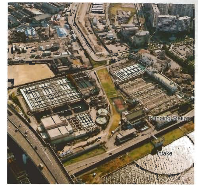
● Shorenjigawa Development (Takami Pumping Station)
