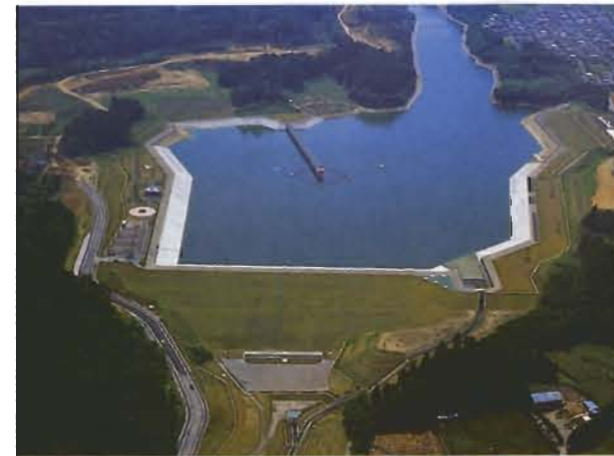
● Boso Canal (Togane Dam)
