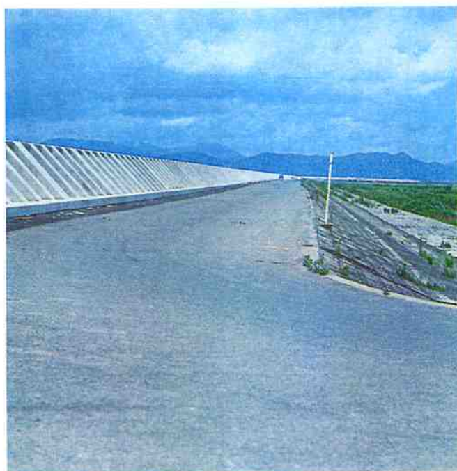
Fig.4-12-2 Higashiyoga Tide-control Bank
