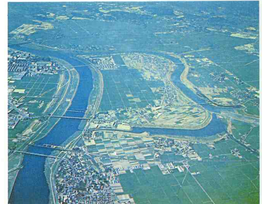
Fig.2-9 Komorino Short-cut (Cut-off) Work
