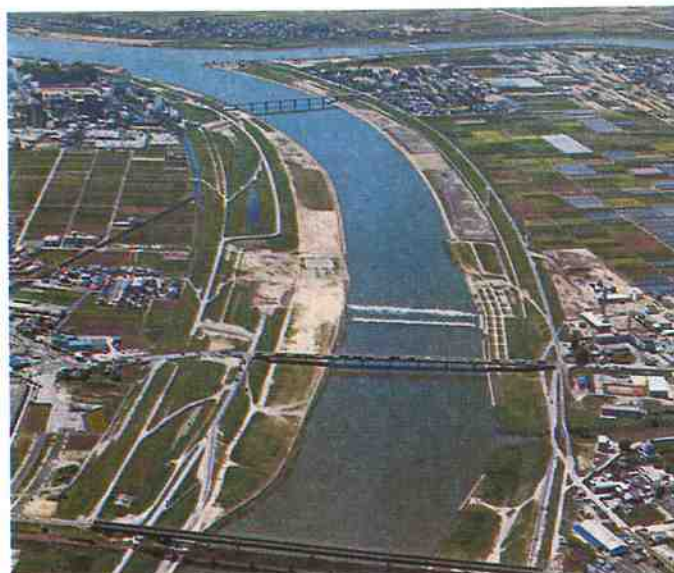
Fig.4-9 Backward Displacement Works of Levee at Higashikushihara
