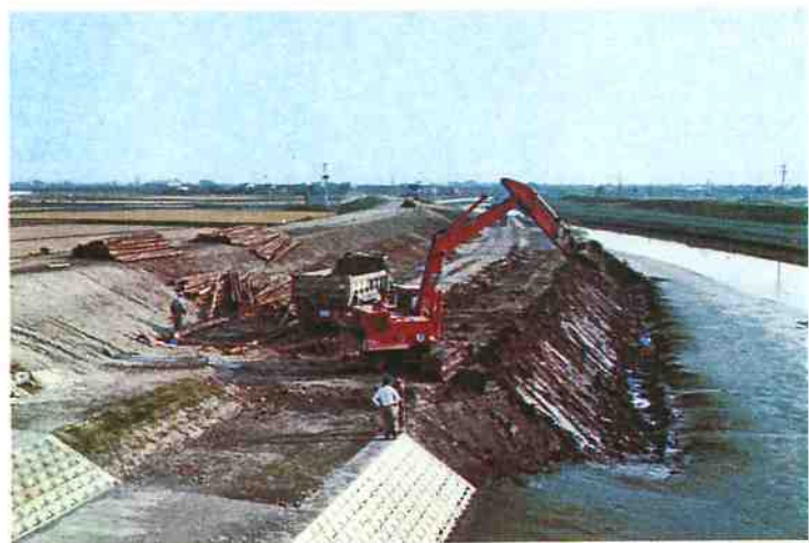
Fig.4-2 Excavation, Banking and Revetment Work in Kojima (Tade River)
