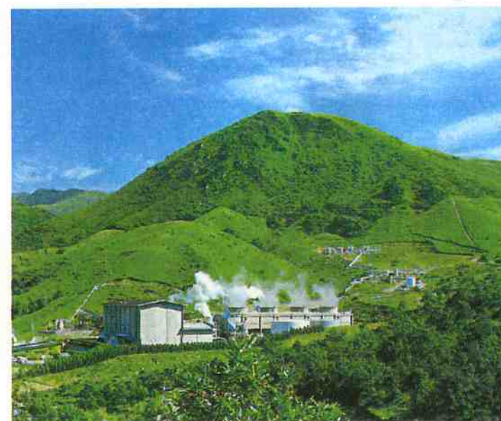
Fig.7-2 Hatchobaru Power Station
