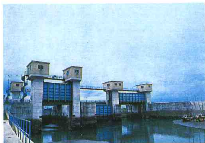
Fig.4-12-1 Hattae Tide-control Gate
