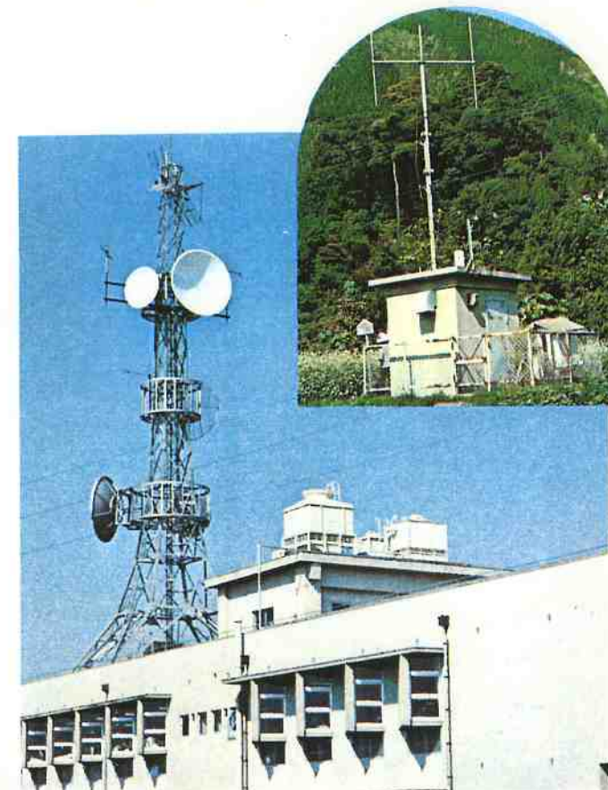
Fig.5-9 Chikugo River Construction Office
