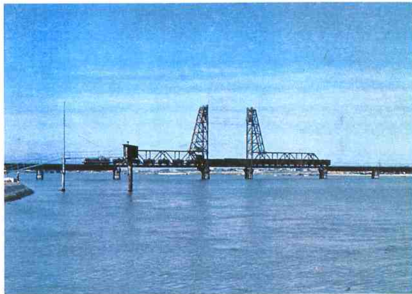
Fig.7-5 Saga-Line Railway Bridge
