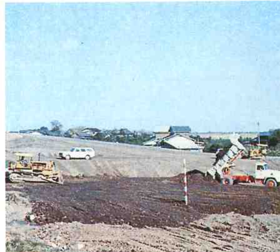
Fig.4-3 Banking Work in Kizuka
