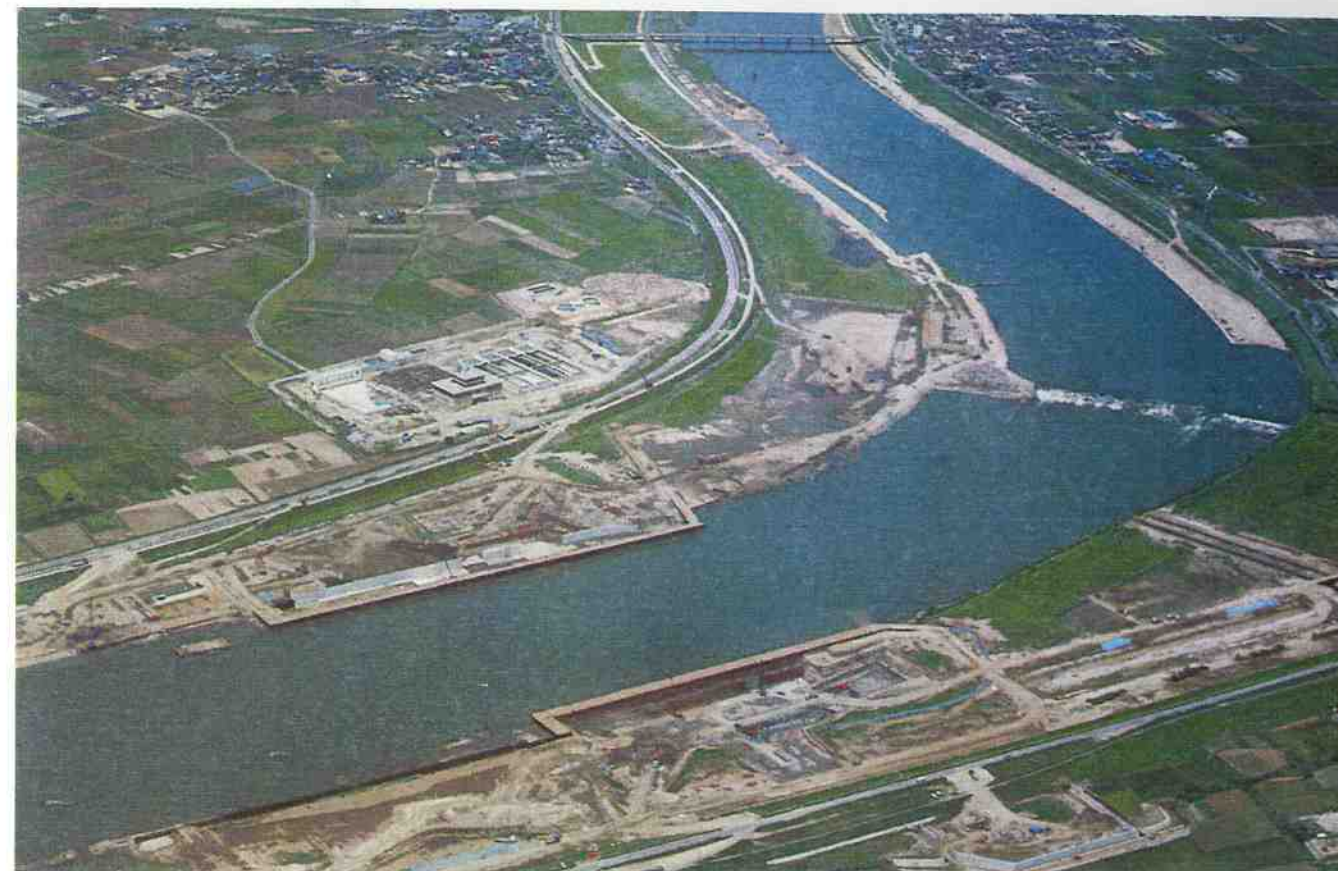
Construction site of Chikugo Great Weir
