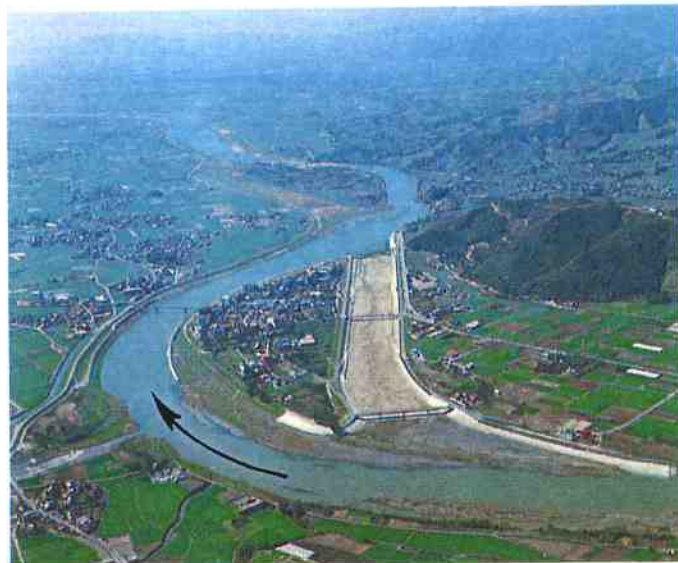
Fig.4-7 Harazuru Diversion Channel
