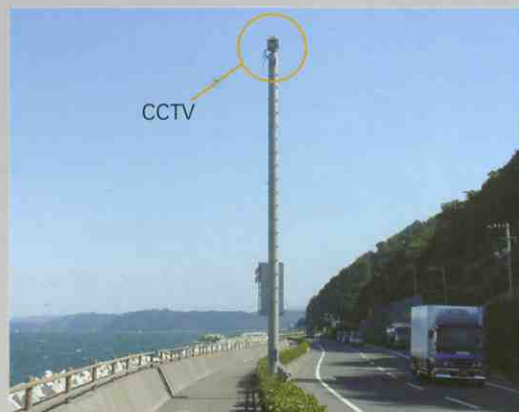
CCTV installed in Kitanada-cho, Naruto City, to mainly monitor surcharges (R11)
