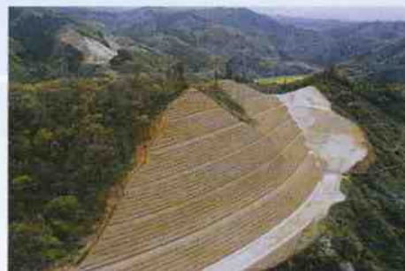
● Construction at Obara Dam
