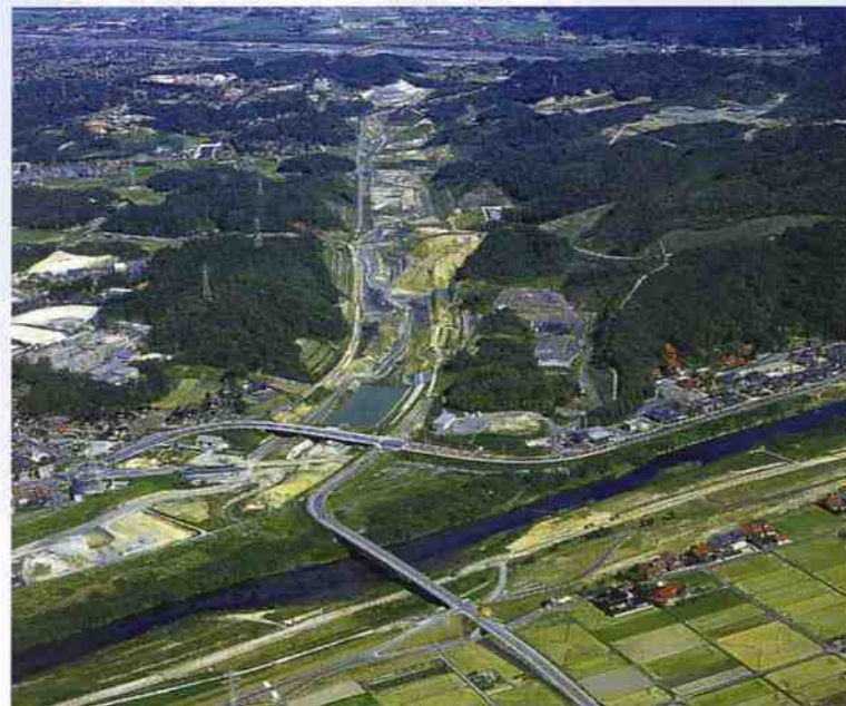
● Construction at Hii River Discharge Channel
