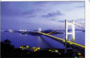
This bridge was opened to traffic in 1988 to link Shikoku and Honshu, Japan's largest land mass. With a total length of 9,368 m, it consists of six bridge sections and four viaducts. The whole route is a double-decker construction, with an expressway running above a railway.
