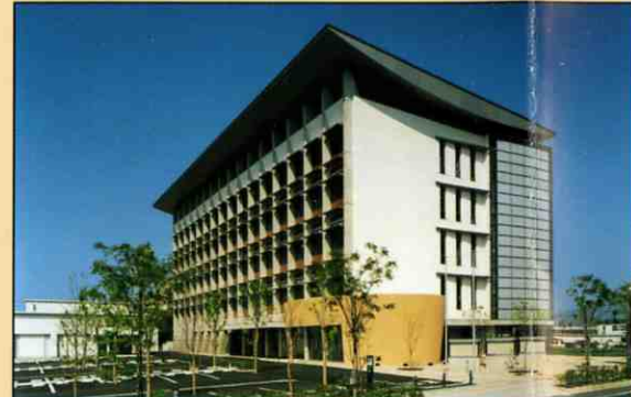
Construction of an eco-friendly government building (Izumo regional government building)
