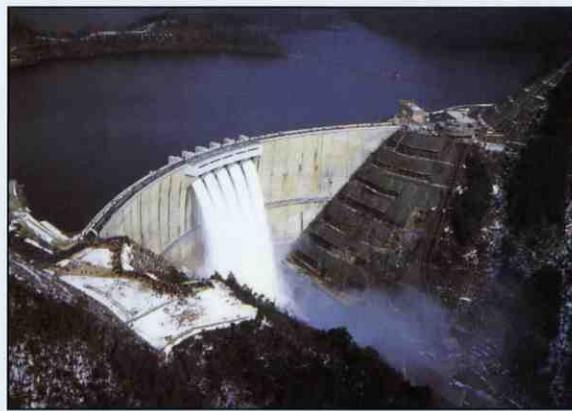
Nukui Dam This dam was constructed for flood control and river flow regulation on the lower reaches of the Otagawa River, and supplies water to 4 cities and 21 towns in Hiroshima Prefecture. This multipurpose dam is the second tallest arch-dam in Japan.
