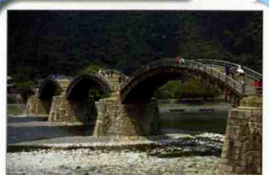
This bridge, regarded as one of the three most famous bridges in Japan, was originally built in 1673. This unique and highly sophisticated five-arched wooden bridge is said to have no negative factors in terms of modern bridge engineering.
