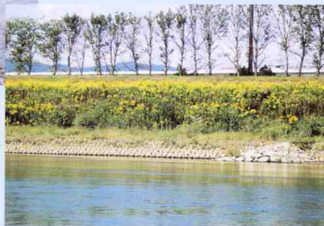
Revetment containing nesting cavities that are river creature friendly fig.9
