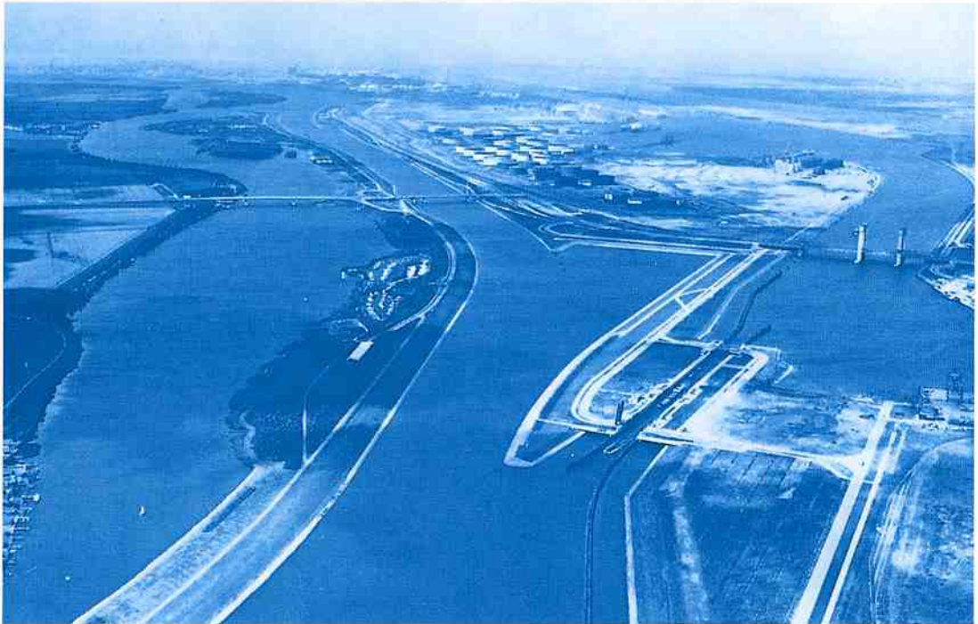
Canal and Lock Gate near Rotterdam, the Netherlands (Photo provided by the Dutch Embassy)
