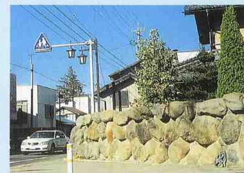
A stone wall is constructed to protect the home from flood damage
