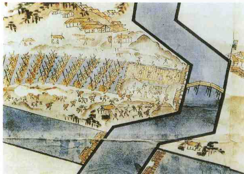
An underground pipe is installed under the Nishi River (inverted siphon)
