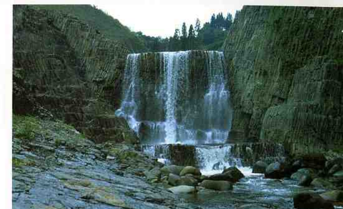
Sabo dam on the downstream Nanatsugama (Nakasato Village) Blocks that look like natural rock are used to build a sabo dam in harmony with the natural environment.
