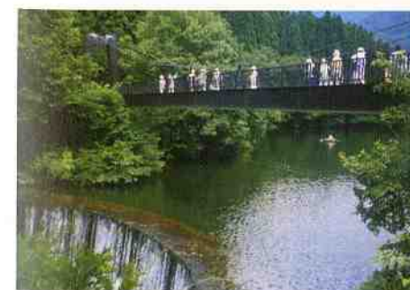
Daigenta River first sabo dam (Yuzawa Town) This is an arch-type sabo dam constructed in 1939.
