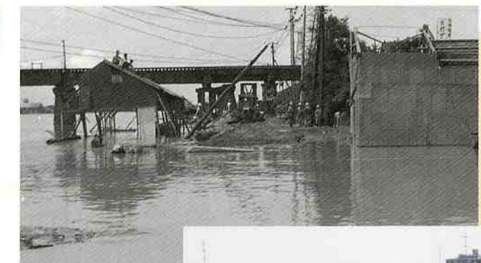
Immediately following Niigata Earthquake, the embankment has been destroyed due to earthquake and tidal wave activity.
