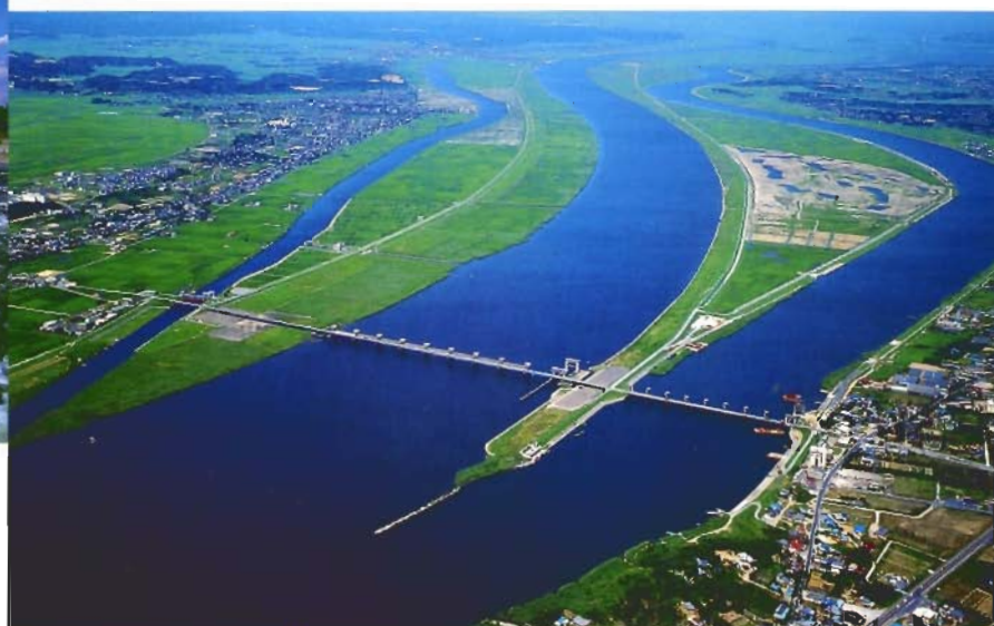
The Tone River Mouth Weir and Hitachigawa Floodgate. Built to curb saline intrusion and supply water. (Tounosho Town, Chiba Prefecture and Hasaki Town, Ibaraki Prefecture) (Photo: Creative ADAC Inc.)
