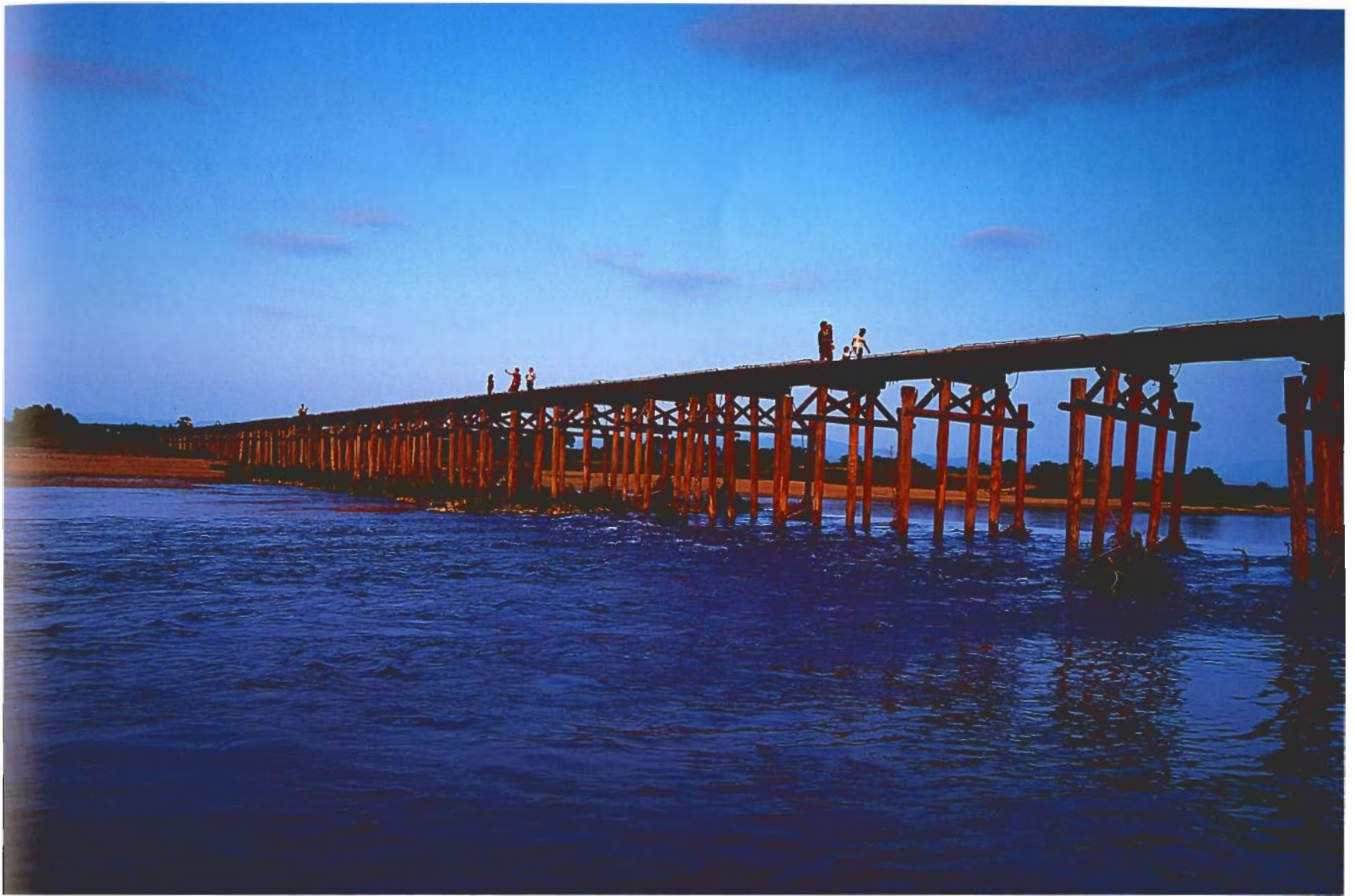
Also known as "Nagarebashi," which means "a bridge that washes out," the bridge was designed to rise off its pillars in times of flooding and float downstream. The wooden bridge is 356.5 meters long and 3 meters wide, and remains standing today as built in 1953. (Kizu River, Kyoto Prefecture) (Photo: Naruaki Onishi/FRONT)
