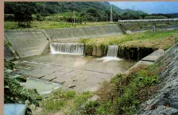
尾白川床固群 (山梨県施工) Ojiragawa Groundsills (by the Yamanashi Prefecture)
