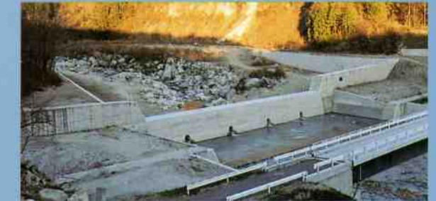
尾白川第三砂防えん堤 Ojiragawa No.3 Sabo Dam 平成元年12月完成。高さ7.5m、長さ146.0mの重力式コンクリートえん堤。 It was completed in Dec., 1989. It is a gravity type concrete sabo dam with 7.5 m of the sabo dam height and 146.0 m in length.
