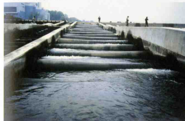
Omaru Irrigation Weir
