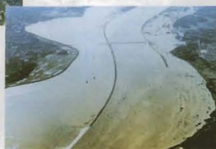
Retention ponds at time of flood
