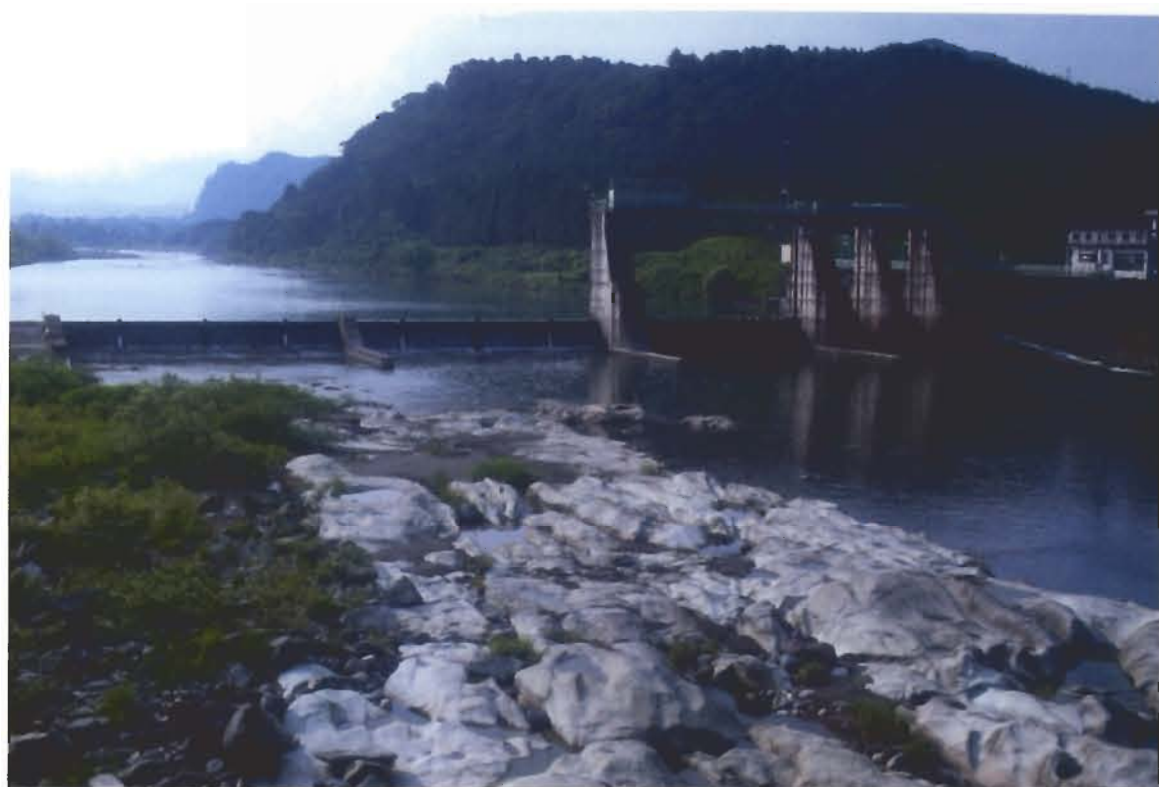
Sanuki head works (Kinu River)
