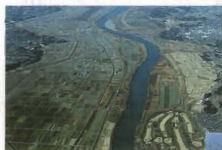
Retention ponds at normal flow (used as agricultural land)
