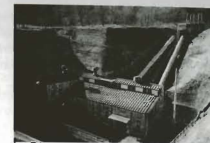
Mukogawara power station
