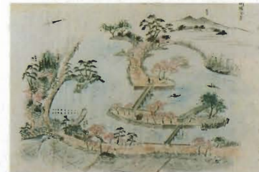
Entire view of the Oka Weir after 1899 sketched by artist Akamatsu Shijiro
