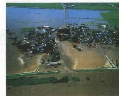
Toyota drainage channel, Ishige Town
