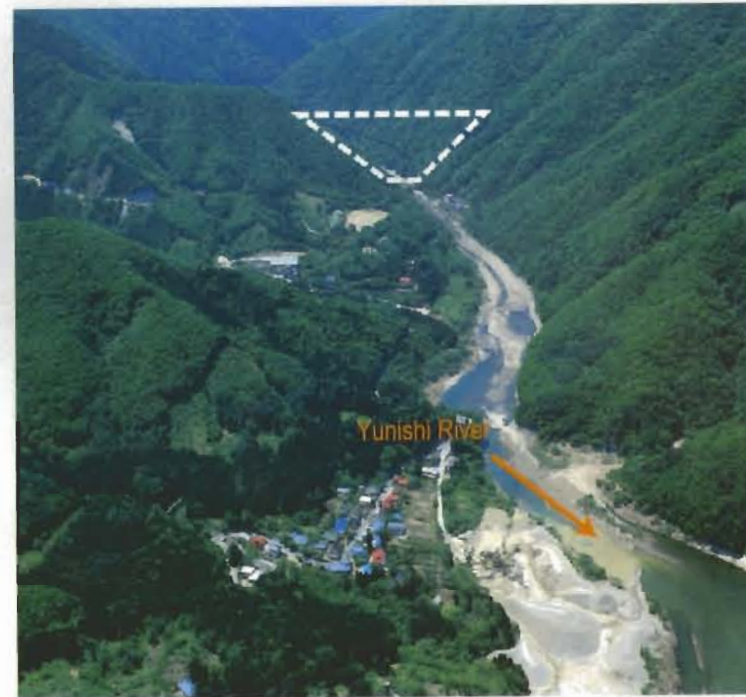
Planned dam construction location
