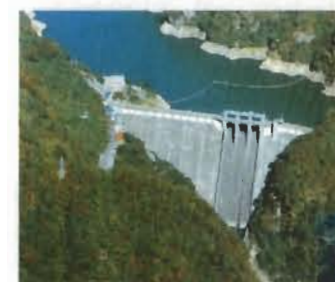
Ikari dam (completed in 1956)
