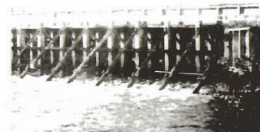
Wooden frame of the Fukuoka Overflow Weir (Constructed in 1896, it was used until 1923)
