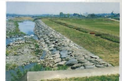
Imaichi channel works with stone laid surface are gently sloped to allow easy access to the river.
