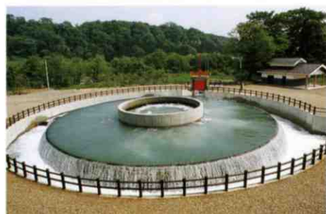
Cylindrical water distribution facility built in 1957 to resolve water disputes involving the Juan and Shigeira weirs. The water is distributed equally by this facility.
