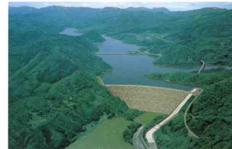
Image of Isawa Dam
