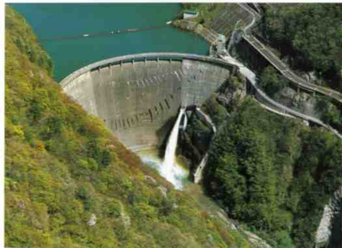
Narugo Dam, the first arch dam designed and built entirely by Japanese engineers
