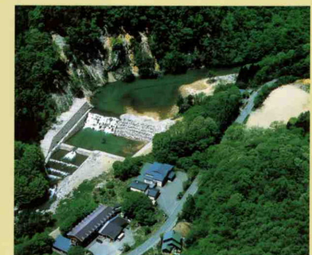
Genbu check dam
