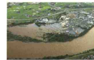
Flooding of Mizusawa Industrial Estate (July 2002)
