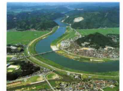
New channel between Yanaizu and Iinokawa
