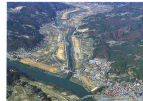
River improvement works for the Satetsu River
