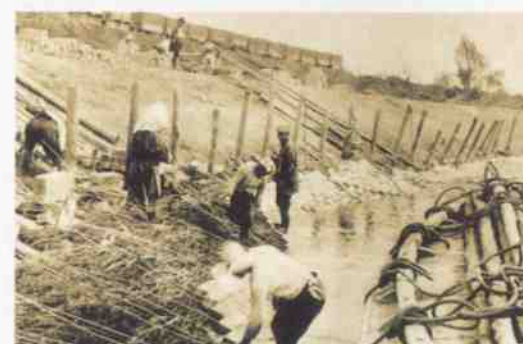
Assembling of the "Okazaki style concrete mattress block" (Ishikari River)
